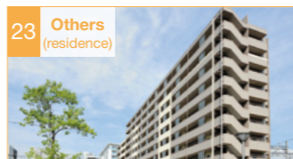
23 Others (residence) Aqualia Chihaya A rental condominium comprised of units mainly for singles and small families to match the local characteristics
