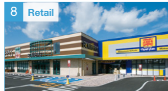
8 Retail Hanahata SC Located in a new residential area and comprising BON REPAS supermarket and Matsumoto Kiyoshi drug store
